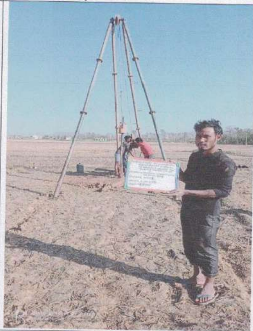
12. Drilling in progress
