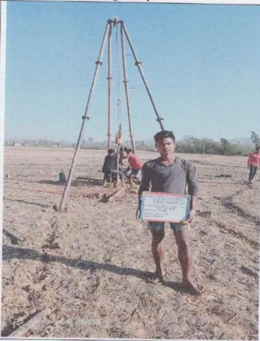
11. Drilling in progress
