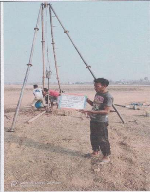
1. Drilling in progress
