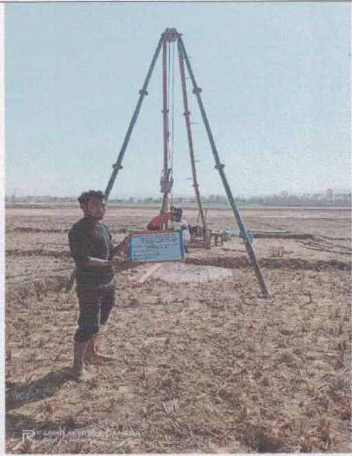
4. Drilling in progress
