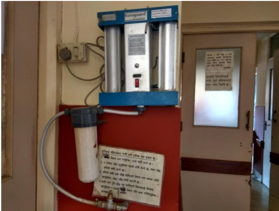
Plate 2-5: Euro guard filter for drinking water Purification
